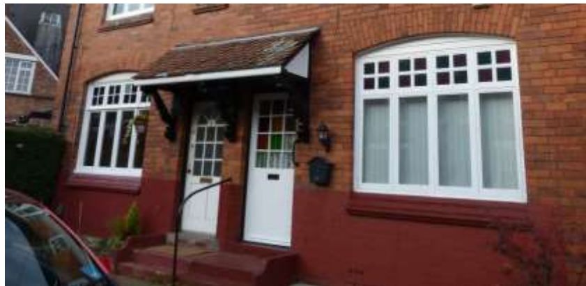
An example of coloured glass in replacement UPVC windows.
