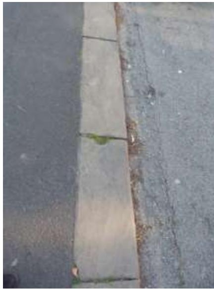
Original kerb stones on Weldon Road
