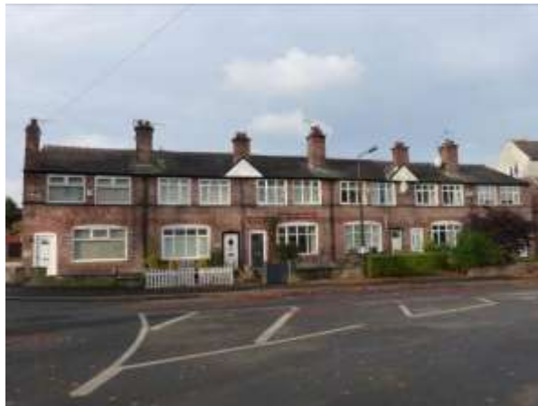
A typical example on Lock Road
