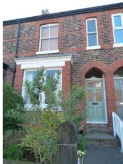
Examples of original style windows and door at No. 24 Weldon Road
