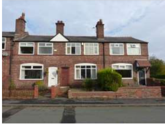
Modern large pane windows on the left and right, with windows of the original proportions in the centre.
