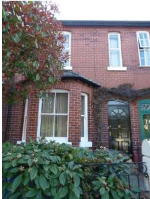
Original style sash windows at No. 12 Weldon Road
