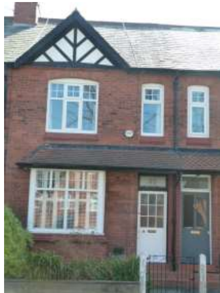
No. 19 Norman Road with original door and replacement uPVC windows in the original style
