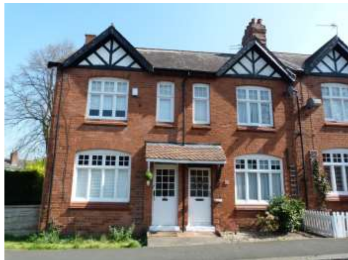
Good examples of surviving windows and doors at Nos. 57 and 59 Lock Road
