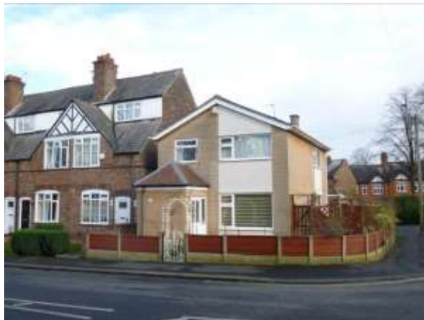
Unsympathetically designed modern housing on Lawrence Road
