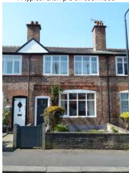
Original window and door at No. 68 Lock Road
