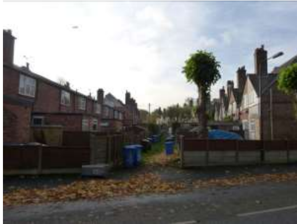
The ginnel between the Lock Road and Lawrence Road terraces.
